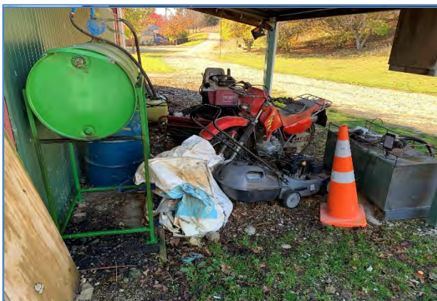
Photo 1: Above ground fuel storage tank and hydrocarbon stains beneath it
