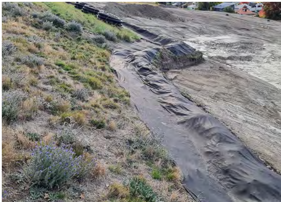
Figure 2: Lined clean water diversion bund on slope (Source: Enviroscope)
