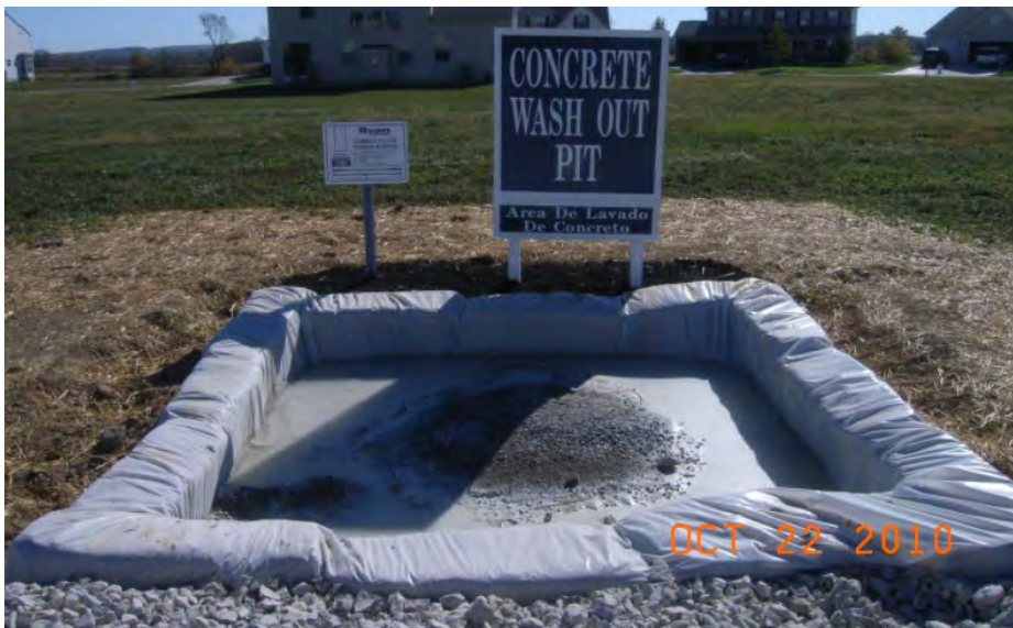
Figure 17: Example of designated concrete wash out pit.
