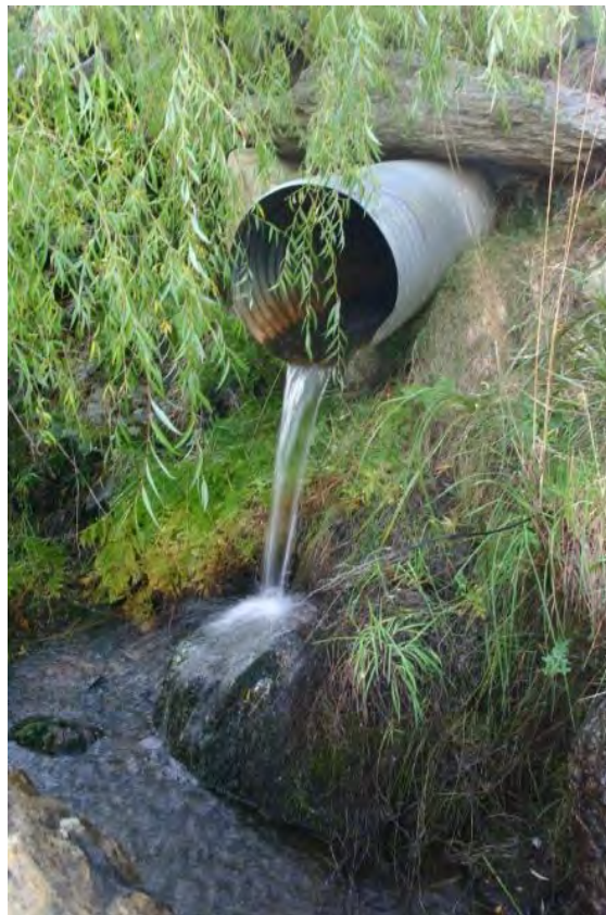
Figure 3. Perched culvert in Pongs Creeks, Cardrona Valley (NZTM 1284323 / 5023115).
