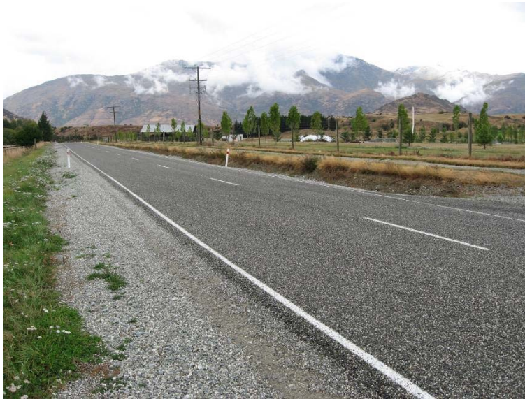
Photograph 4: McDonnell Road, Looking South at Existing Golf Course Entrance
