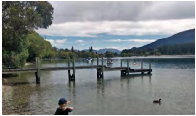
Figure 2 – Existing Jetty #S14C
