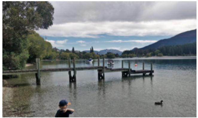
Figure 2 – Existing Jetty #S14C
