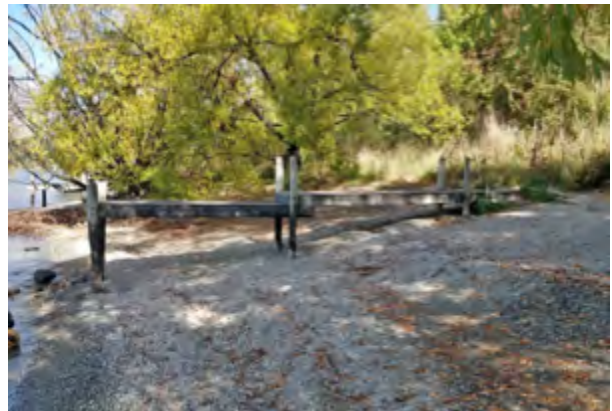
Figure 2 – Existing Jetty #S97
