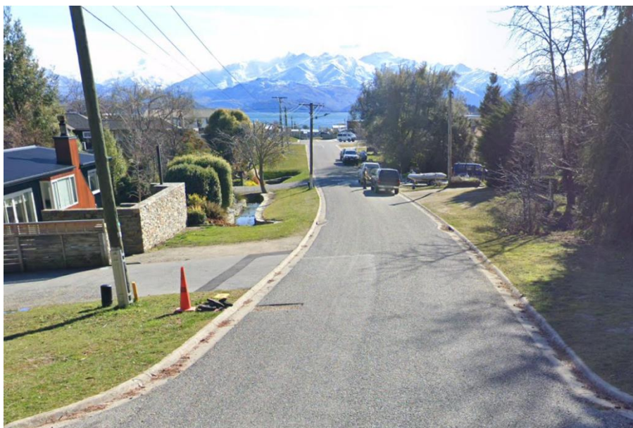
Photograph 1: Youghal Street Looking North (Site on Left)
