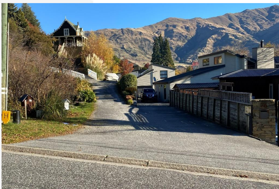
Photograph 2: Property Driveway (Site on Left)
