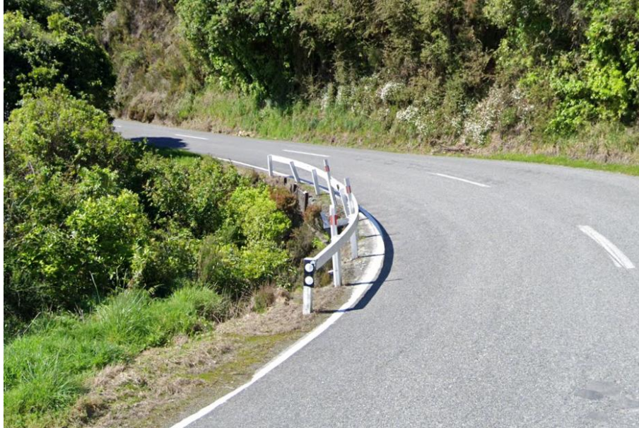
Photograph 11: Example of Fencing to Deter Drivers from Steep Drop-Off
