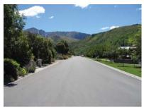
Try to avoid excessively wide carriageway with low profile kerb and channel.
