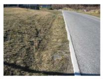
Adopt grass drainage swale and flush concrete edge to seal. Instead place concrete beneath seal edge.
