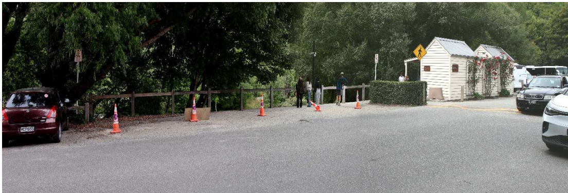
Figure 15: Temporary Bus Stop Position (marked by cones and barely visible signage, no pavement markings indicating a bus stop)
