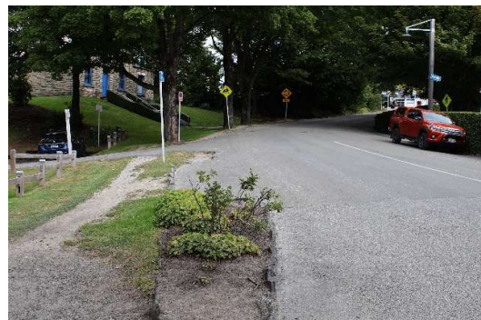
Figure 27: Shoulder formation outside library site.
