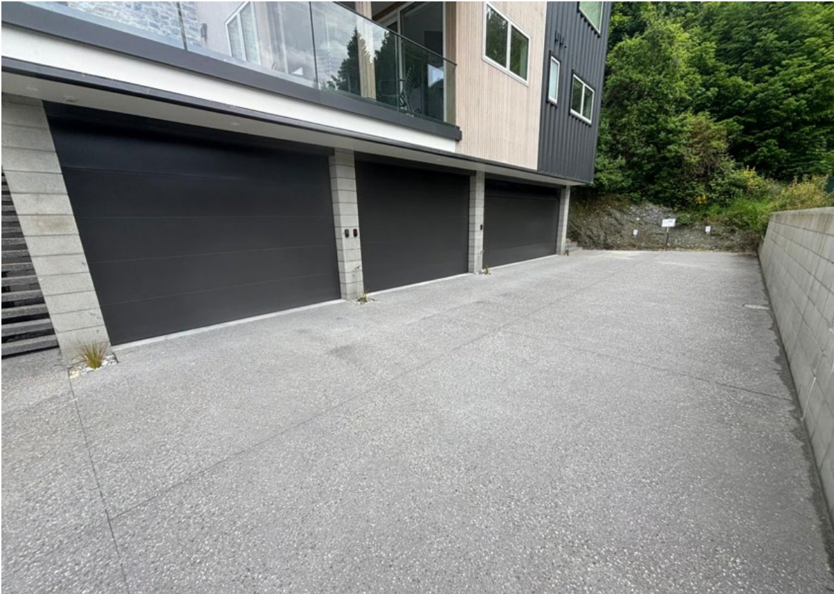
Figure 4: Parking for 10B and 10C (Source: Site Visit)
