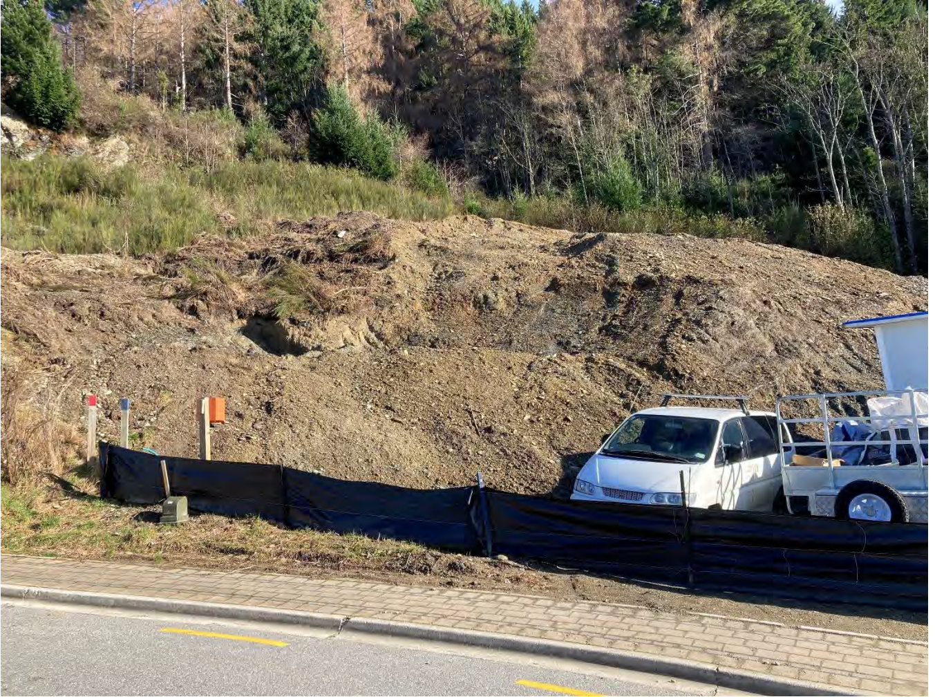
Photo 1: Looking northwest across the property. Two rock exposures can be seen and are where structural measurements were recorded.
