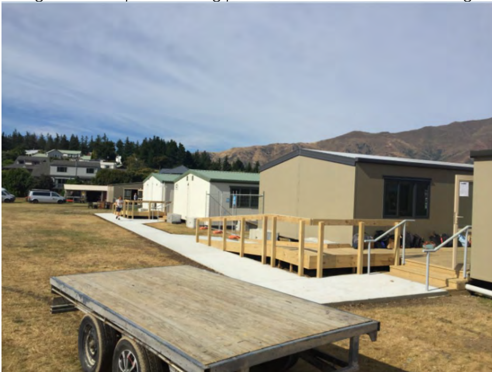
Figure 4: Example of existing portacom classrooms and decking
