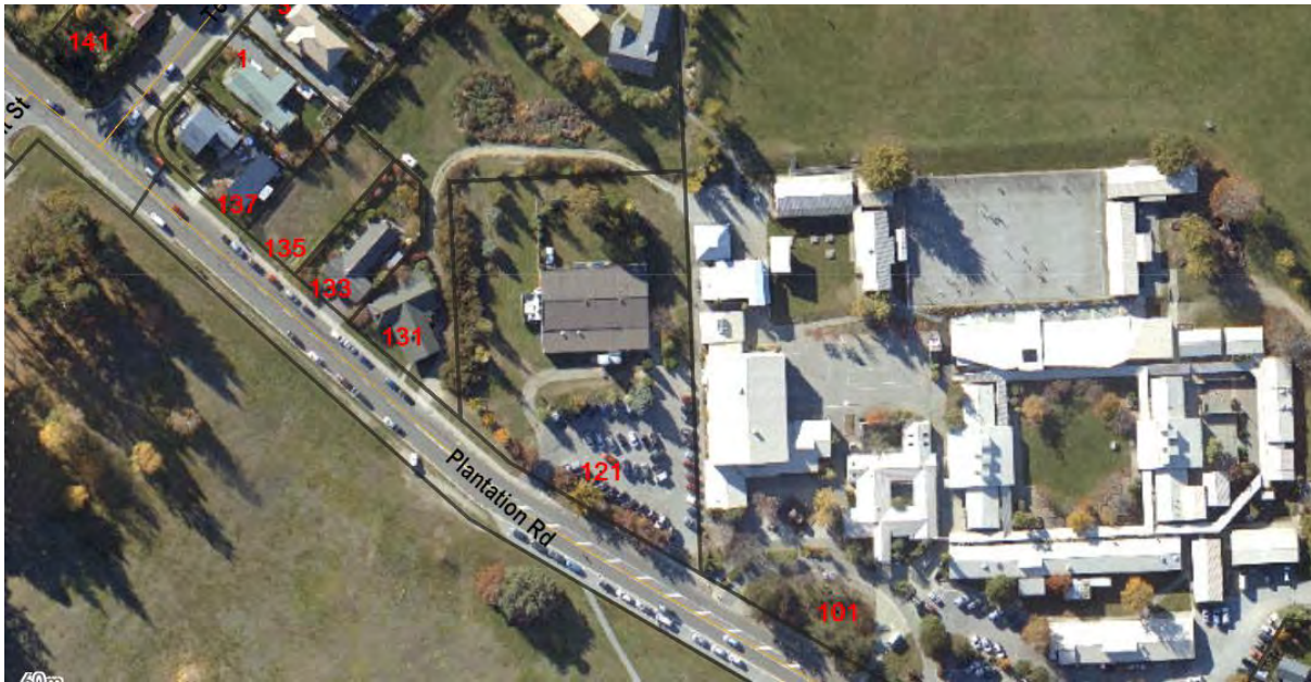
Figure 1: Aerial view of the subject site (121 Plantation Road) and Mt Aspiring College to the east
