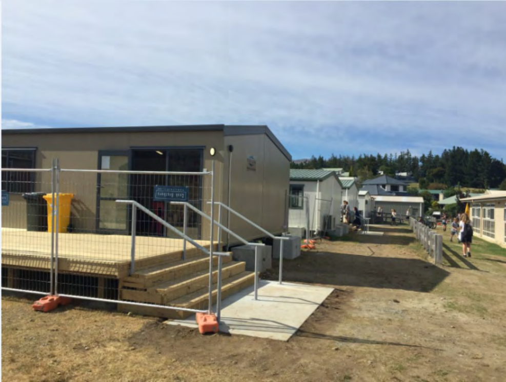
Figure 3: Example of existing portacom classrooms and decking
