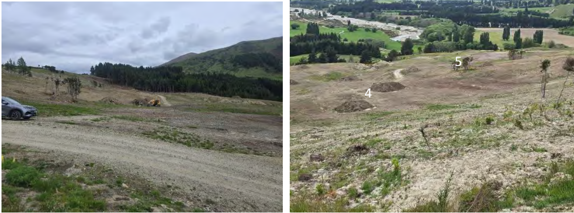
Photo 1: View of rear scarp from east side of landslide.
