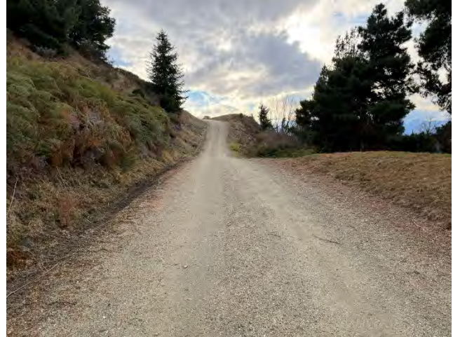
Established conifers and a sporadic bracken present along the lower portions of the existing access track
