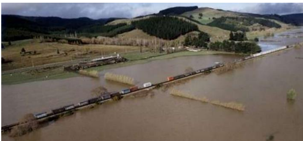
Figure 6-11: South Island Main Trunk Line after 2006 flood on the Taieri Plains, (Otago Regional Council, 2013).
