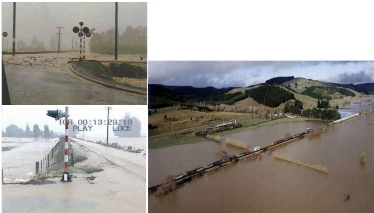
Figure 7-19: Taieri Gorge Railway (left) and South Island Main Trunk (right) inundated by flood waters in the April 2006 floods (Goldsmith et al., 2015; O’Sullivan et al., 2013).
