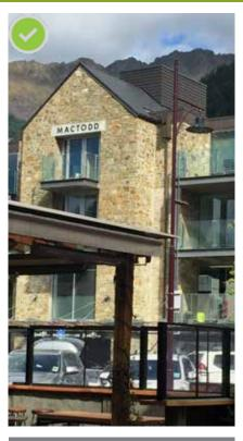
Varying materials and modulation in the building facade can create visual interest as well as reducing the perceived visual mass of a building. A balance of glazing with solid materials is recommended to provide a human-scale feel to buildings. The provision of balconies is a simple solution to create modulation as well as provide outdoor living space amenity for occupants. Plant equipment is also screened from the street.
