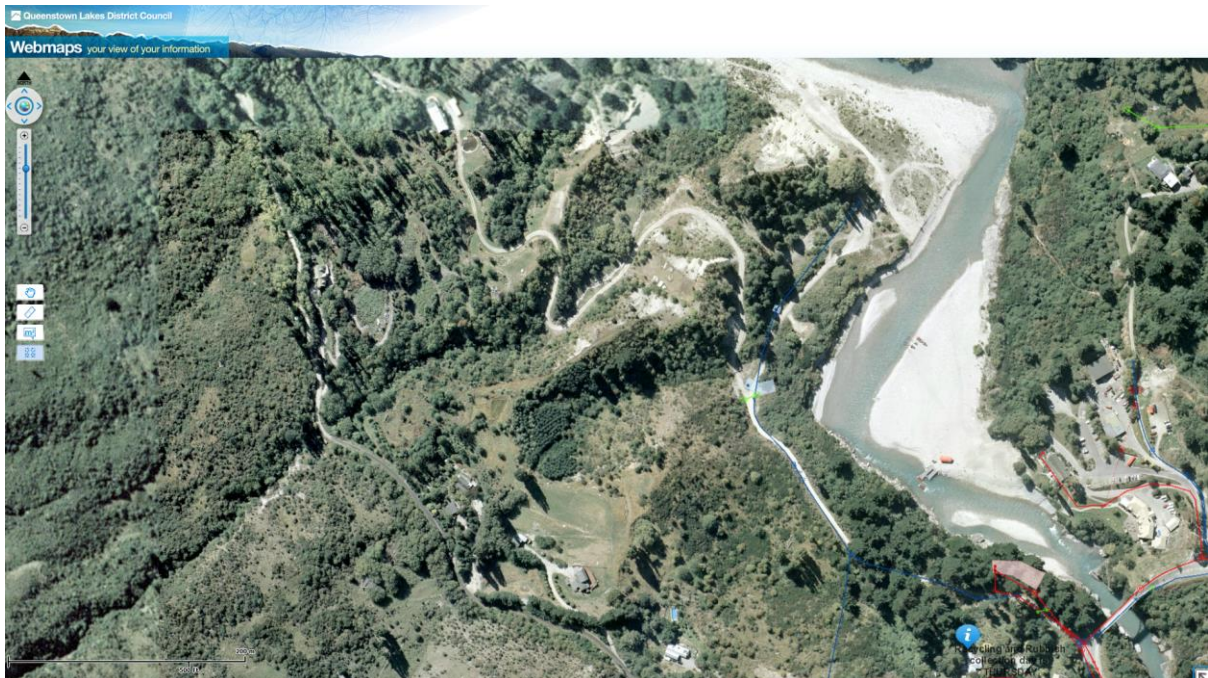
Figure 1 –Bores and Pump Station shown in Blue adjacent to dog leg in Shotover River. Source – QLDC Website 09.03.15
