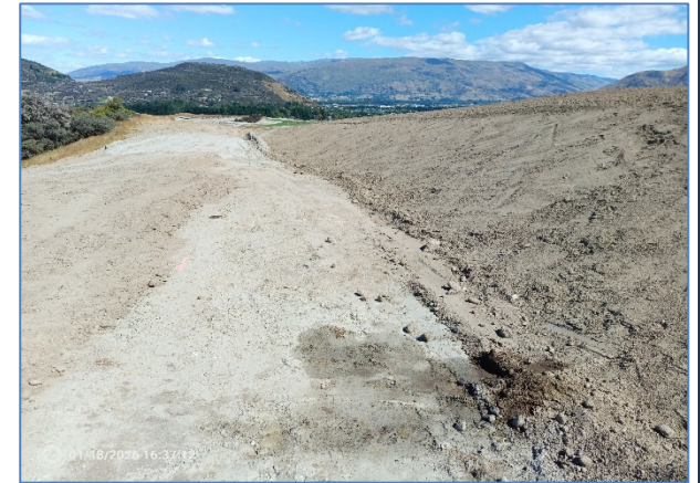
Photo 3: South western portion of the site, showing a small fuel spill.
