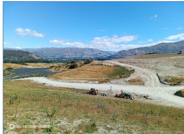
Photo 2: Western-central portion of the site, viewed from the north west facing south east.
