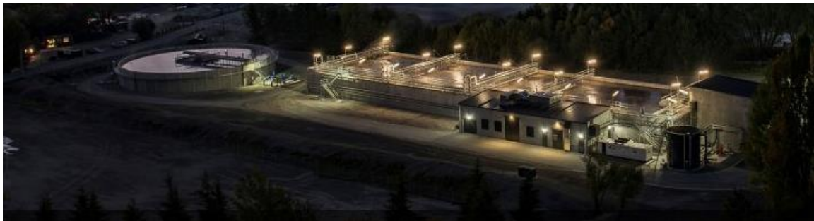
Figure 1: Phot of the Shotover Wastewater Treatment Plant in Queenstown. Sourced from http://www.eis.co.nz/projects/shotover-waste-water-treatment-plant-queenstown-nz
