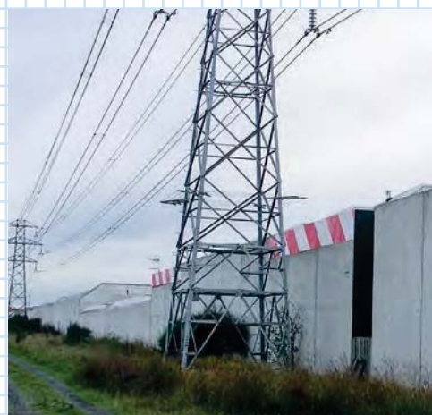
Building has been built too close to lines in violation of NZECP 34 requirements.
