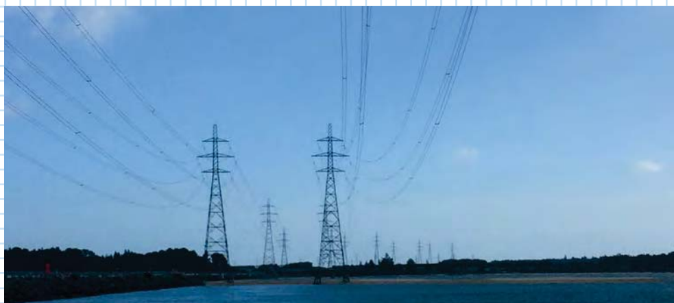
Even moderate winds show just how much the conductors (wires) can swing from the centreline of a transmission line.
