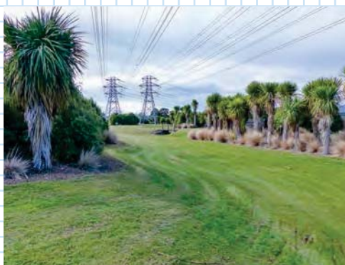
Screening using plants is an effective way to minimise the prominence of transmission towers.
