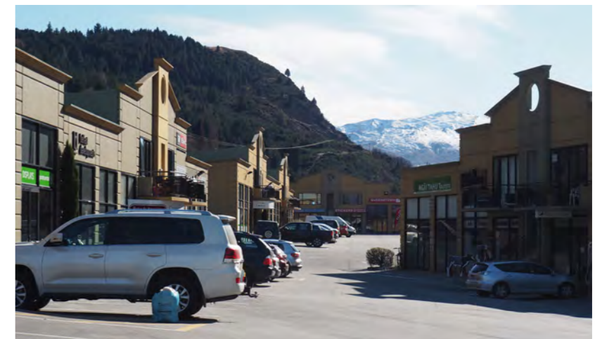
View North towards the commercial internal frontages and carpark of the Gorge Centre. Coronet Peak in background
