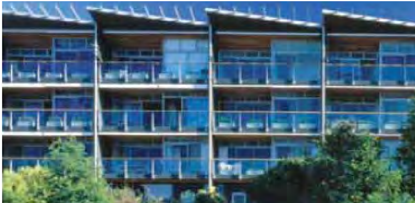
Figure 66: Balconies in built form
