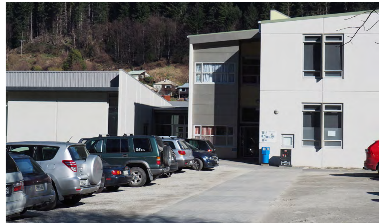
View West to taller school buildings on Northern edge of site
