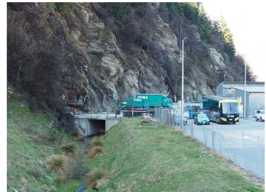
Northern extent of Horne Creek Culvert
