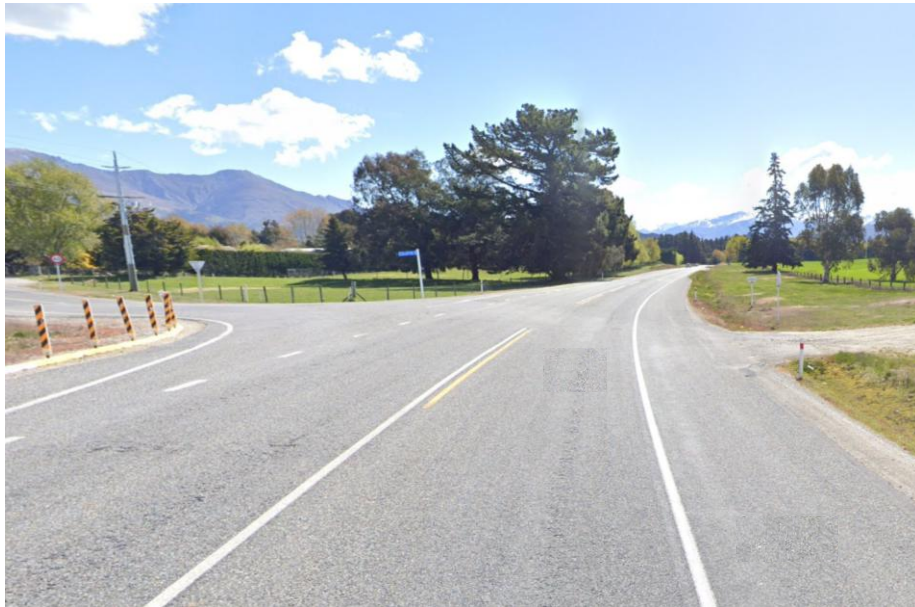
Photograph 6: State Highway 6 / Ballantyne Road Intersection Looking West
