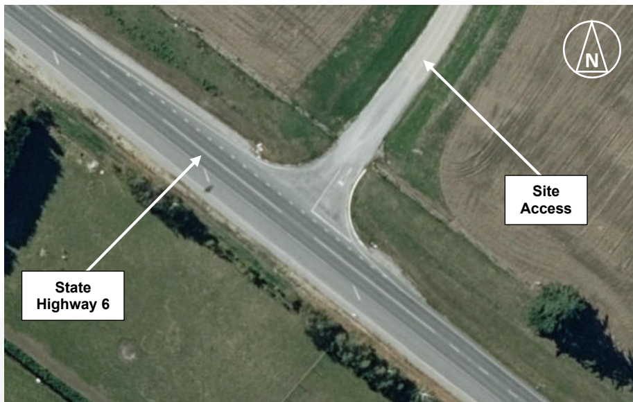
Photograph 3: Aerial Photograph of Existing Access into Site Showing Widening
